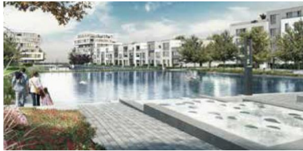
52 Grad Nord, Berlin (under construction)
