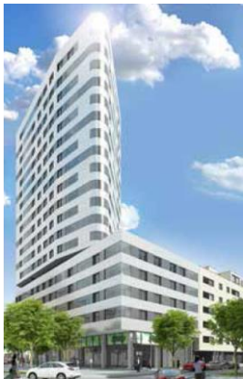
Skytower, Vienna (under construction)
